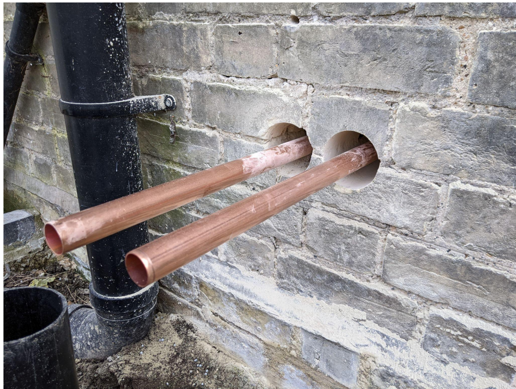
Pipes through wall
