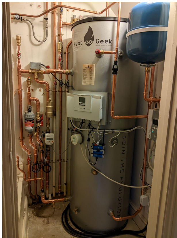
New 230L tank - mains pressure
