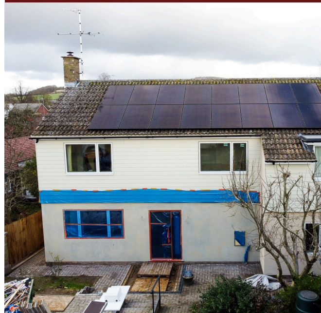
Works in progress
