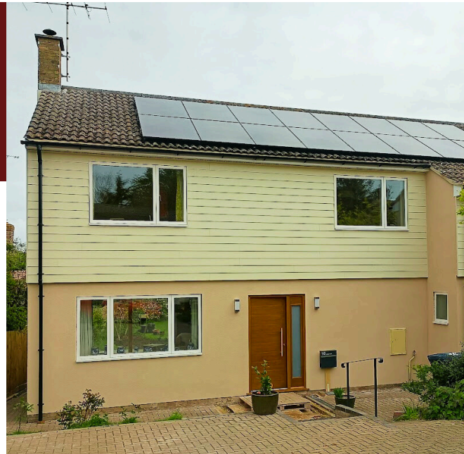
External wall insulation & solar PV
