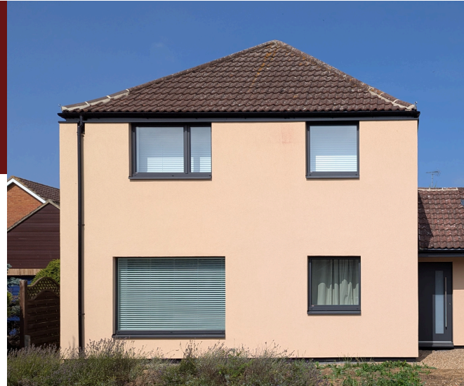
External wall insulation to front of property
