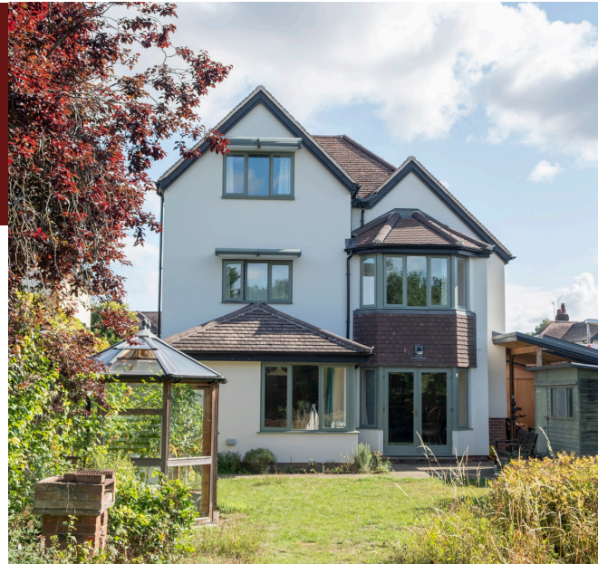
Rear of house with external wall insulation
