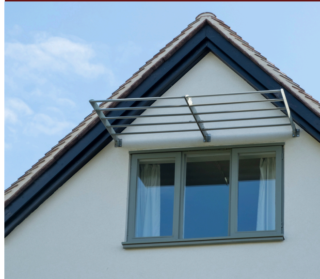
Solar shading with brise soleil
