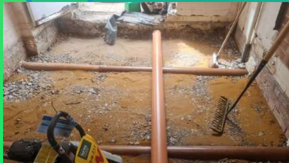
Below concrete slab: vent pipes for susp floor running under direct vent pipe for wood stove
