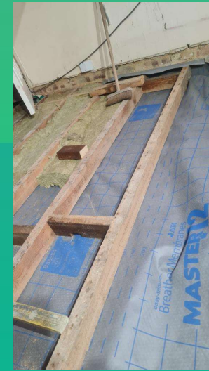
Kitchen floorboards lifted to insulate
