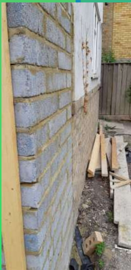
New wall: chose masonry lined with old for EWI
