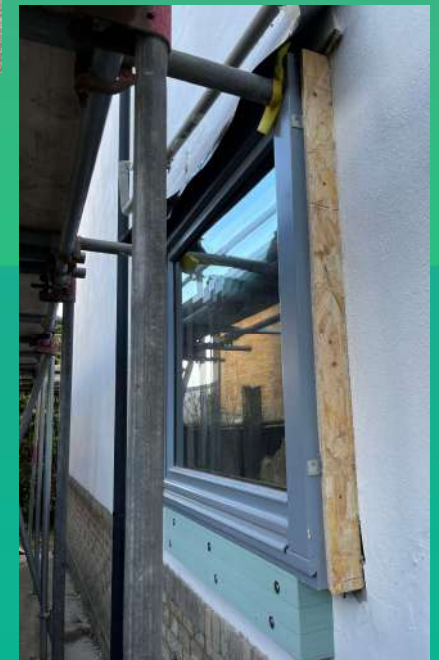
Structural insulation - Partel Alma Vert – from recycled bottles
