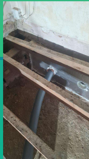
Service penetrations made airtight
