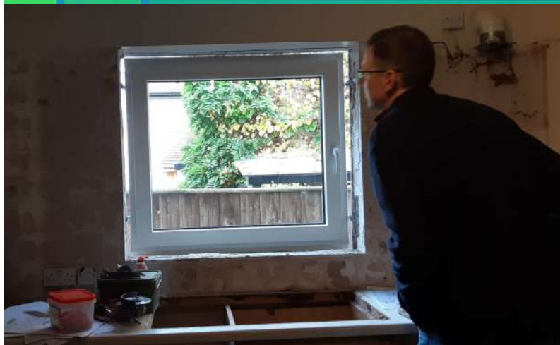
Trial window installed w Struct Insulation in External Wall insulation zone
