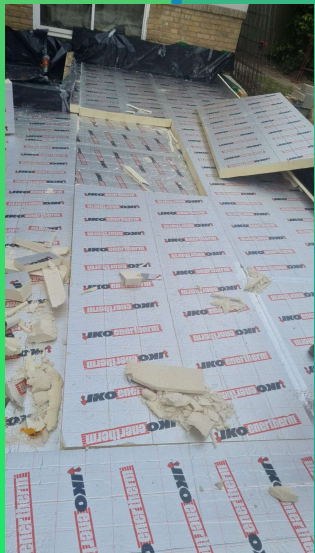
New SunRm solid fl 250mm IKO Enertherm PIR insulation
