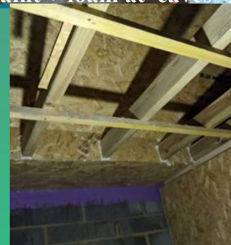
New bedrms roof: tape, OSB Zero, AT paint + foam at eaves
