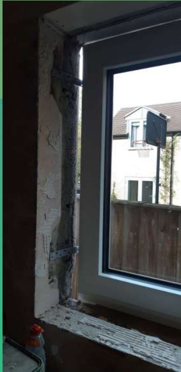
Trial window installed w Struct Insulation in External Wall insulation zone
