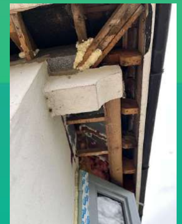
More insulation added to eaves
