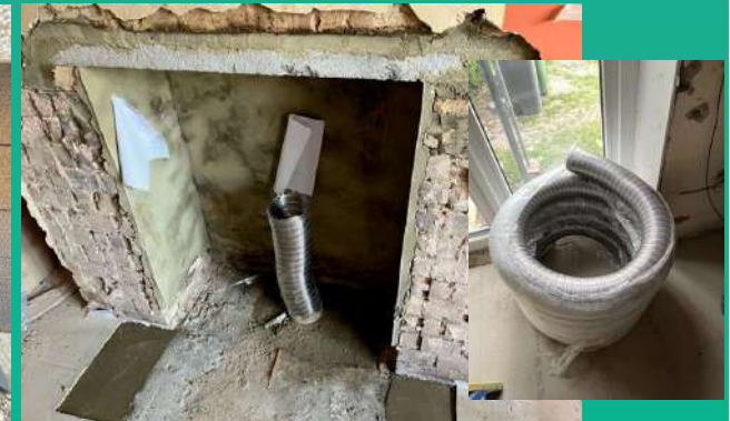
Direct vent airtight hearth connection
