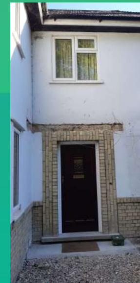
Front concrete canopy removed
