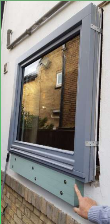
Trial window installed w Struct Insulation in External Wall insulation zone
