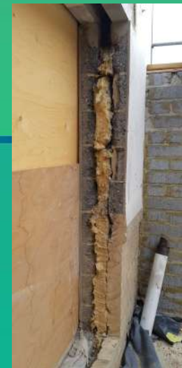
Some exist cavity wall insulation; void to be closed
