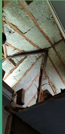
Loft roof: 50 Rockwool Flexi ( \lambda = 0.035 ) + 150 PIR Celotex ( \lambda = 0.022 ) + airtight OSB
