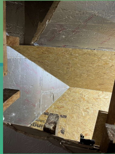
Loft roof: 50 Rockwool Flexi ( \lambda = 0.035 ) + 150 PIR Celotex ( \lambda = 0.022 ) + airtight OSB
