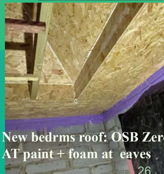
Bedrm 3 exist roof: tape, OSB Zero, AT paint + foam at eaves
