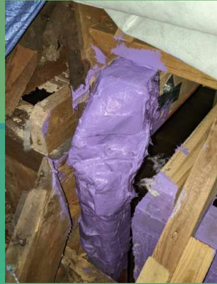
New bedrms roof: fibrous AT paint on steel chimney bracing
