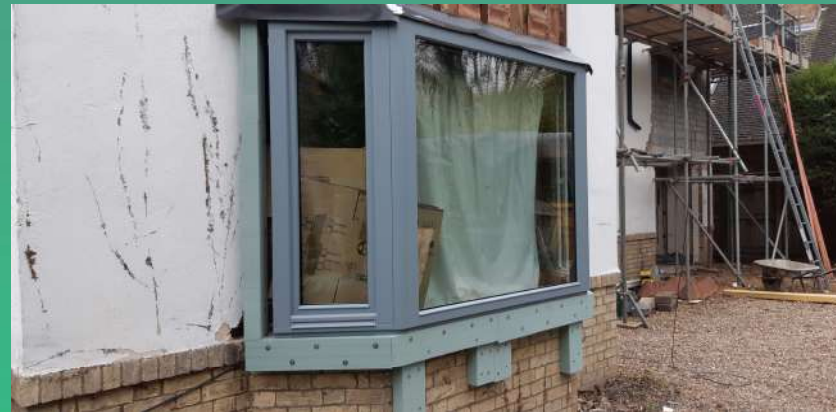
Structural Insulation supporting windows in External Wall insulation zone, temporary rain covers
