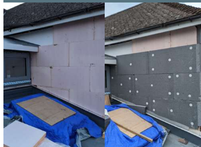
External wall insulation
