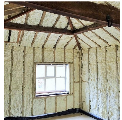
Spray foam insulation
