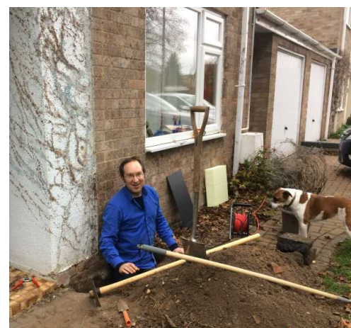
Preparing the groundworks
