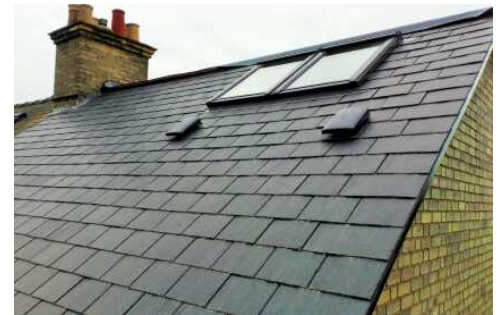
MVHR intake & extract vents
