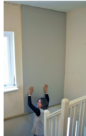
Gill holding up insulated plasterboard
