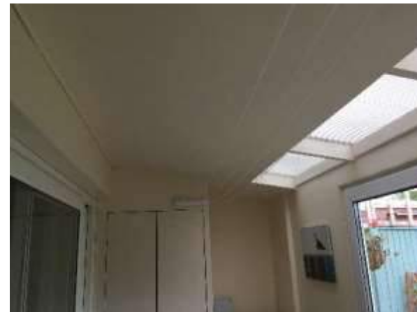
Insulation on ceiling and pipes to left
