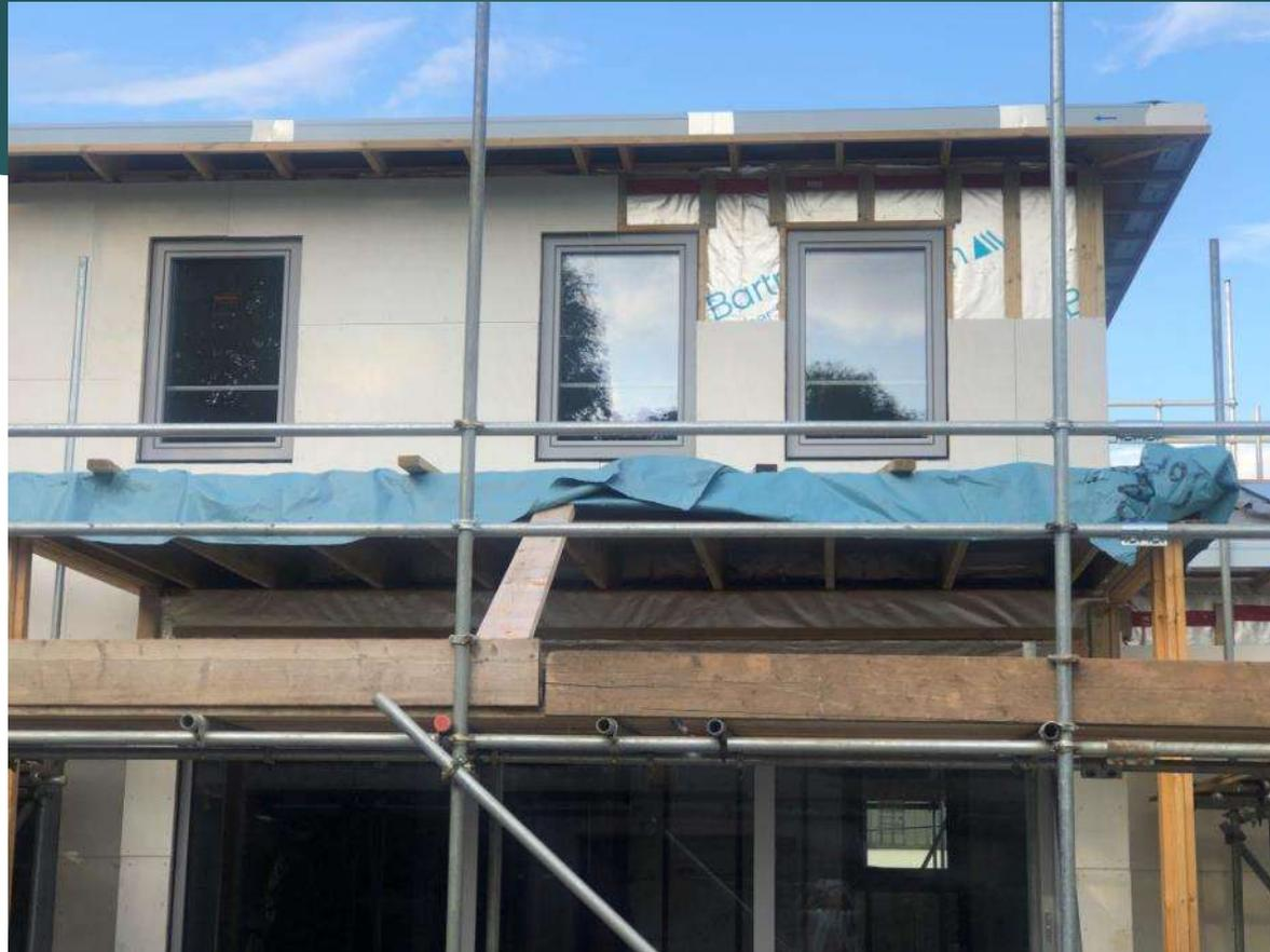
**The accuracy of the timber frame fabrication allowed the ordering of the windows and doors before the start of the build.**
