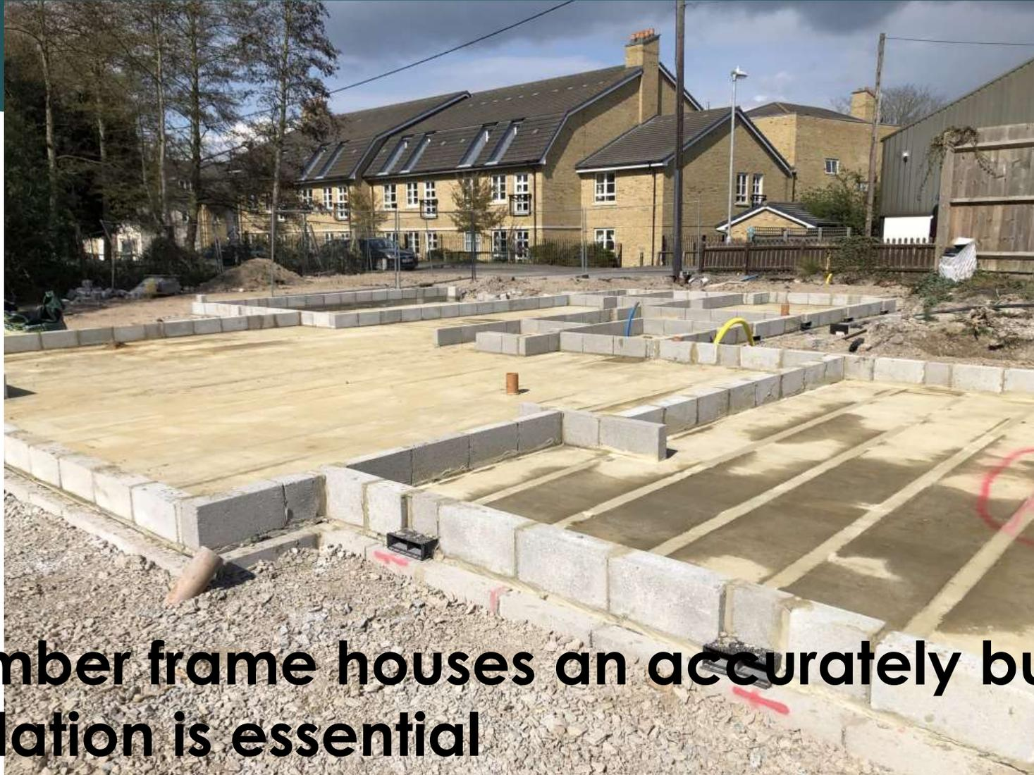
**For timber frame houses an accurately built foundation is essential**
