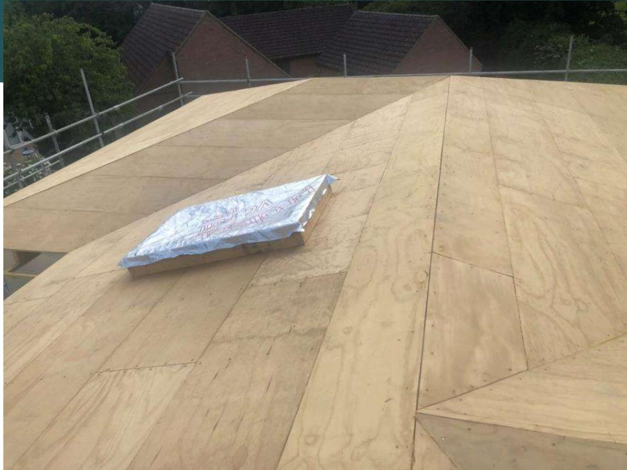
**We chose to fully sark the roof which helped with insulation and airtightness work**
