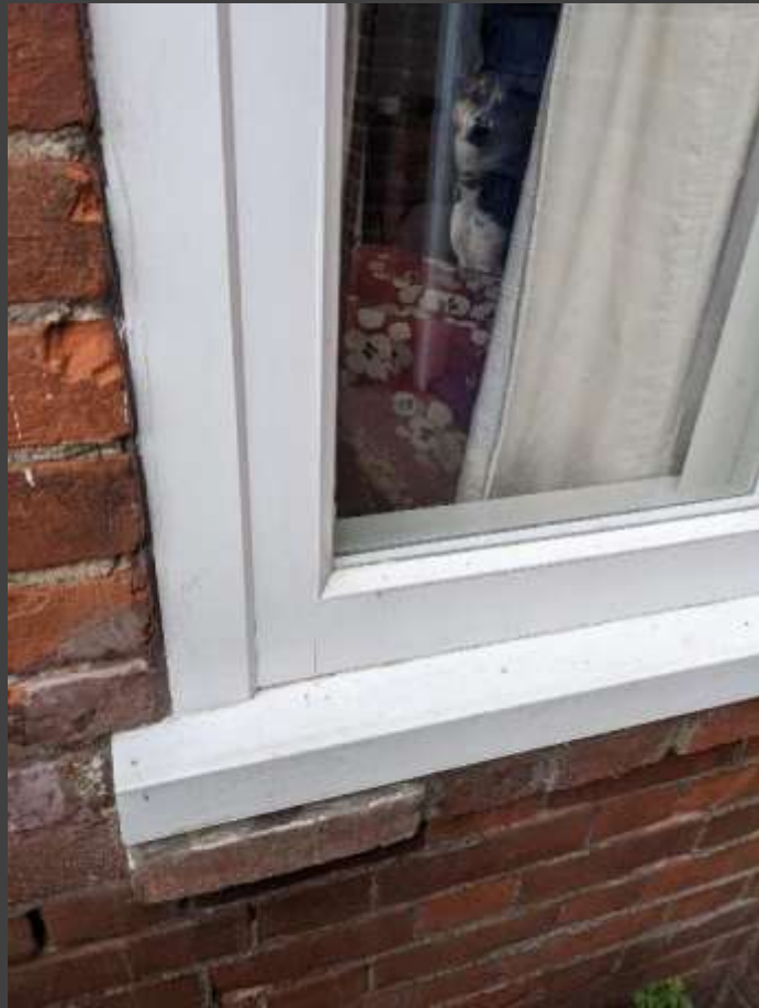
Strengthening and cladding with Tricoya
