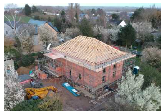
Rockwool-filled extruded clay blocks
