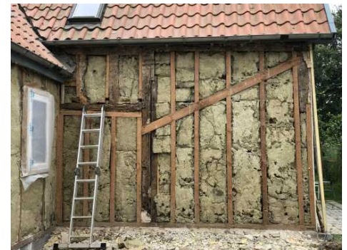
Adding 150mm wall insulation, 2022
