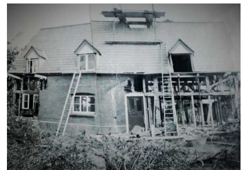
Removing brick facing, 1984
