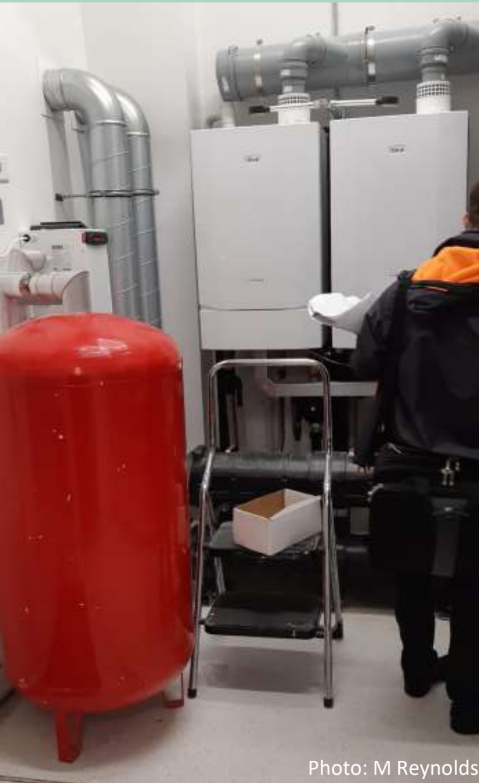
Church & Halls site: Efficient gas boilers
