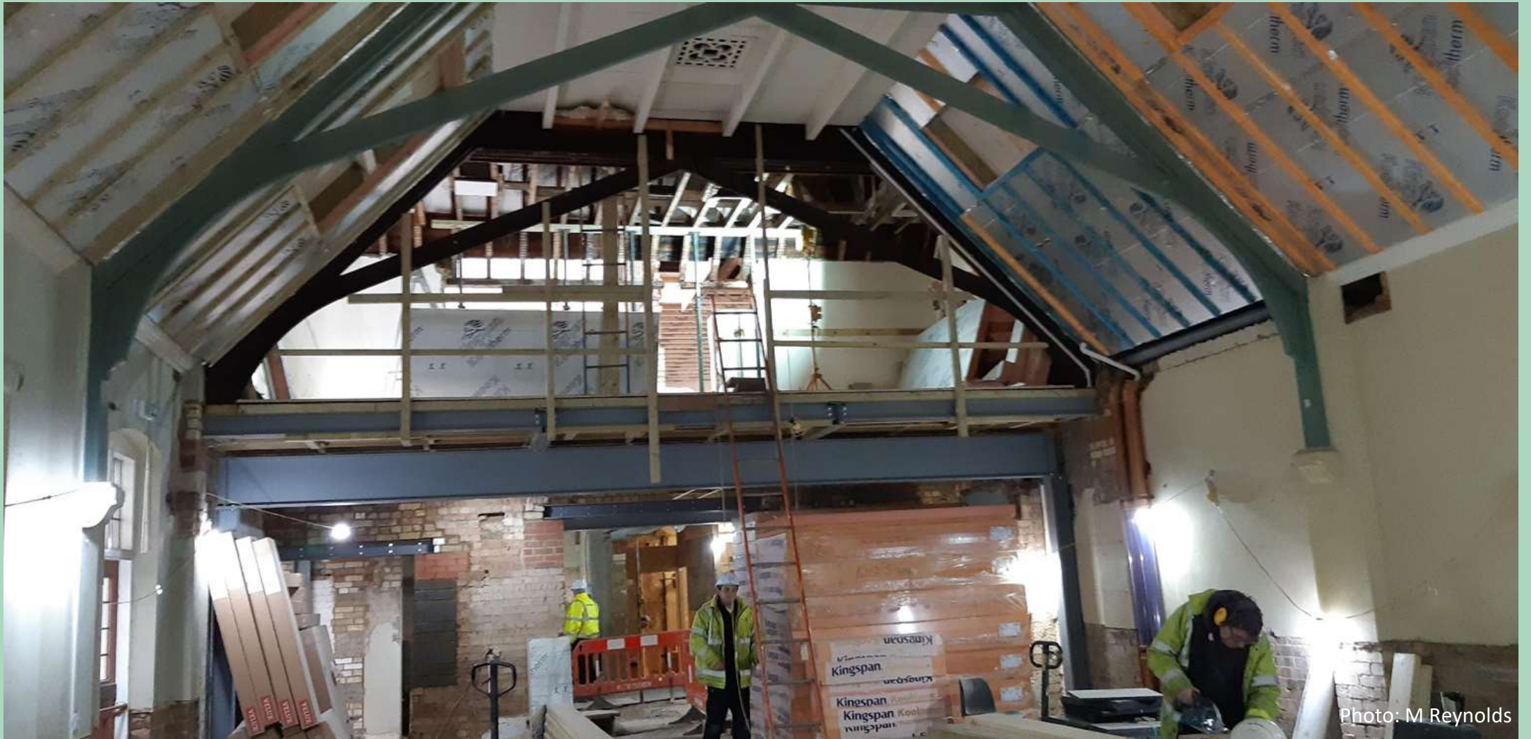
Gibson Hall roof insulation
