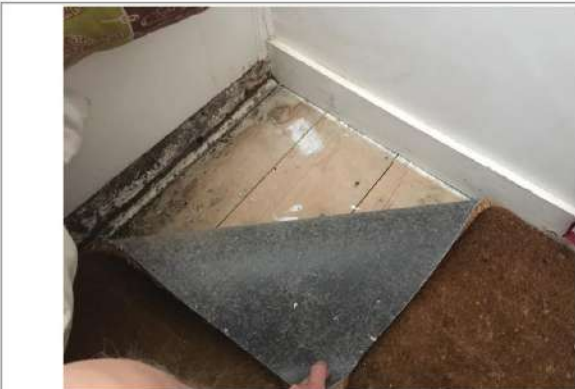
Living Room: The floor in the entranceway leaks air through the cracks, this could be sealed with silicone caulk. The flap for the letterbox also does not seal very effectively.
