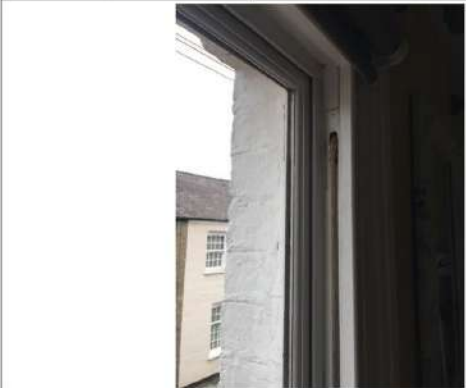
Front Bedroom: Air enters through a crack around the outside edge of the window, goes into the sash boxes and then comes into the room around the pulley.
