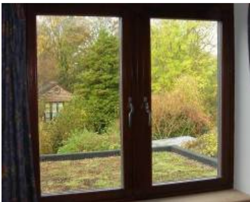
A newly-laid sedum roof in Gwydir St
