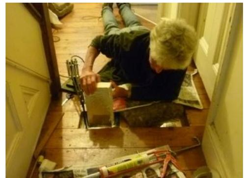
As backup, I hammered a nail partially into each joist to hold up the celotex. In some places, I could hammer a wedge on top of the sleeper wall, to wedge the sheet up against the underside of the floor boards.
