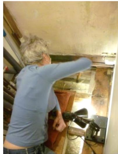
Putting the last block of celotex into position, before replacing the floor board.
