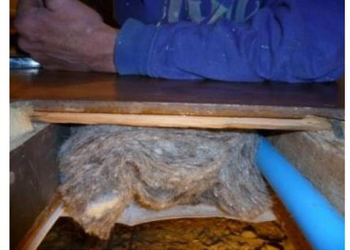
To maximise its performance in reducing air leakage, I glued the tyvek to the walls at the sides.
