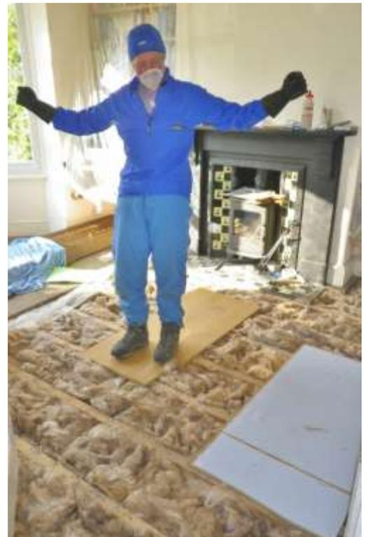
We also used one small roll of [homeECO Insulation](#), made from recycled PET bottles: unlike glass-fibre, it can be handled without irritation and so is good for filling tricky gaps or insulating from below the floorboards. It's extremely hard to saw widths from the roll, but otherwise is easy to handle and to tear into appropriate strips.
